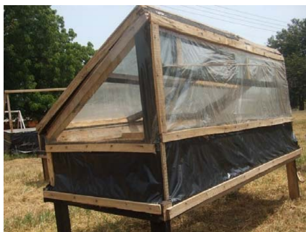
Figure-3. Panel C with black polythene sheet lining the exterior of the drying platform.
