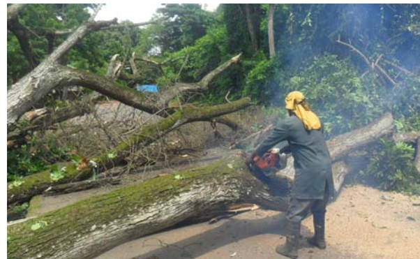
Figure-4. Cross-cutting a felled tree to clear the site.
