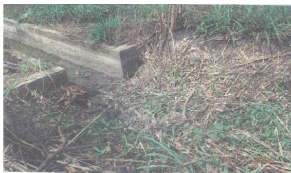
Figure-1. Heavily silted Sata scheme canal.
