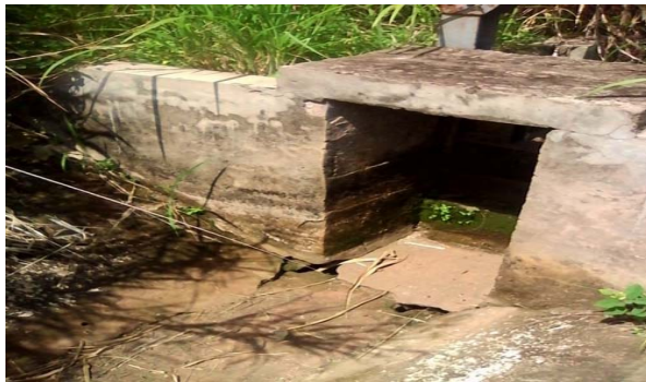
Figure-7. One of the numerous cracks on canal floor 5 years after rehabilitation.
