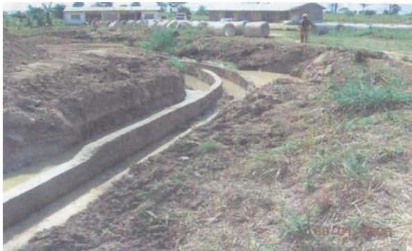
Figure-2. Sataso Scheme canals under reconstruction (2009).
