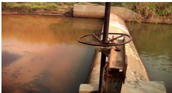
Figure-3. The rehabilitated weir with greater intake capacity.
