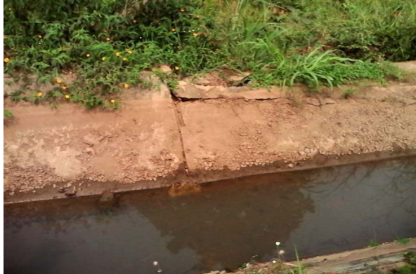
Figure-8. Low water level in canal due to serious seepage.
