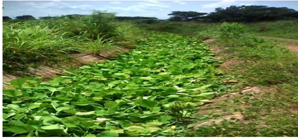
Figure-6. Silted and weed infested main canal at the Sataso Irrigation scheme.
