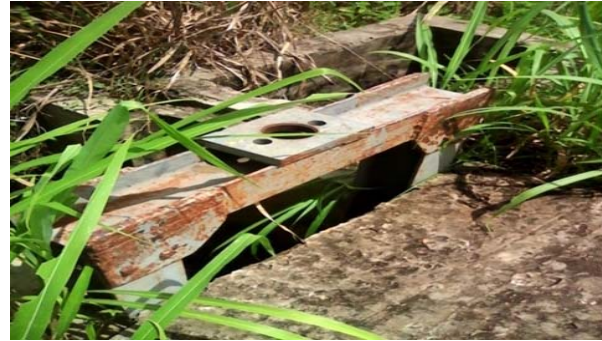
Figure-10. Non- functional check gate.
