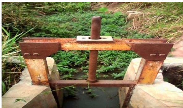
Figure-9. A turnout gate without a gate and driving wheel to control water levels.
