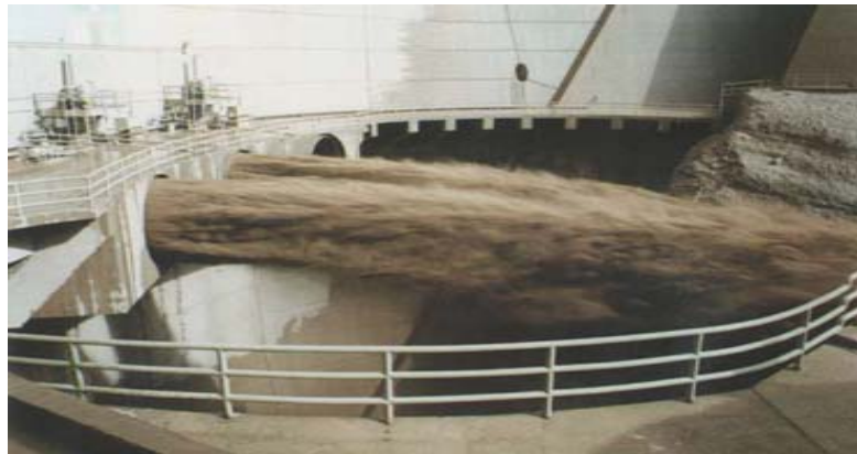
Figure-2. The outlets after the opening ( Dez Reservoir, Iran).
