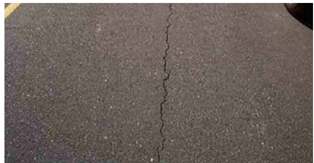
Figure-2. Longitude crack repair by crack sealing and crack filling [5].
