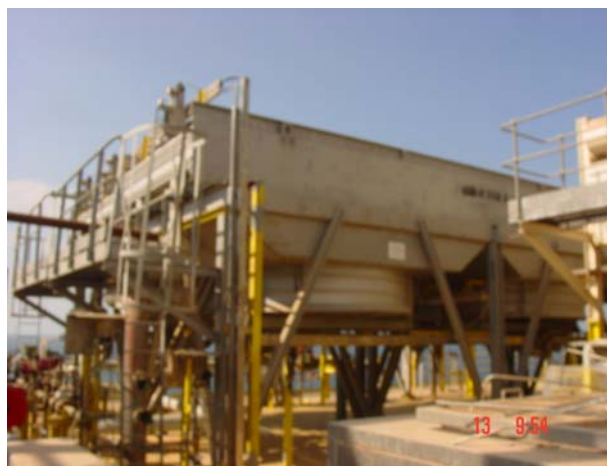
Figure-1. General view of air cooled heat exchanger, the tube bundles are on top and the fans are inside the plenum.
