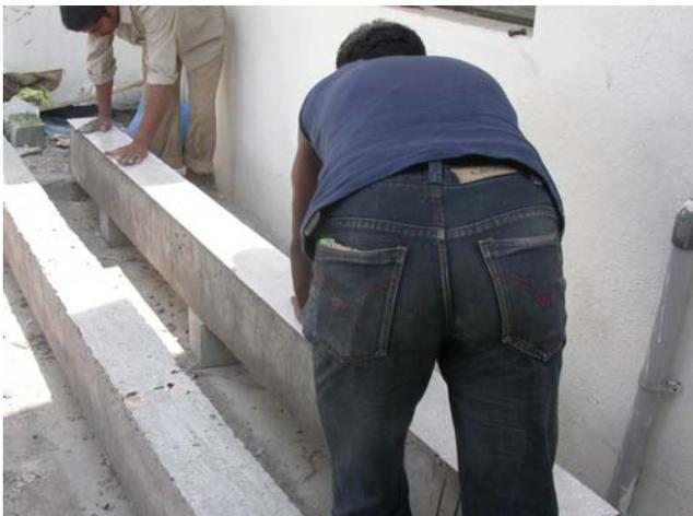
**Figure-1.** Bonding GFRP plate using adhesive.
