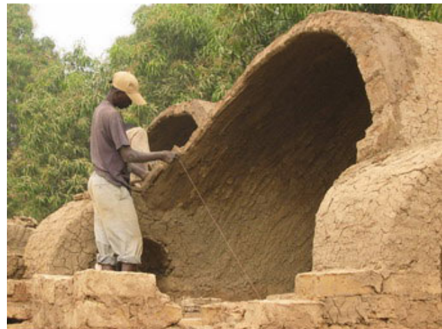
Figure-1. Nubian vault building process in Burkina Faso [6].
