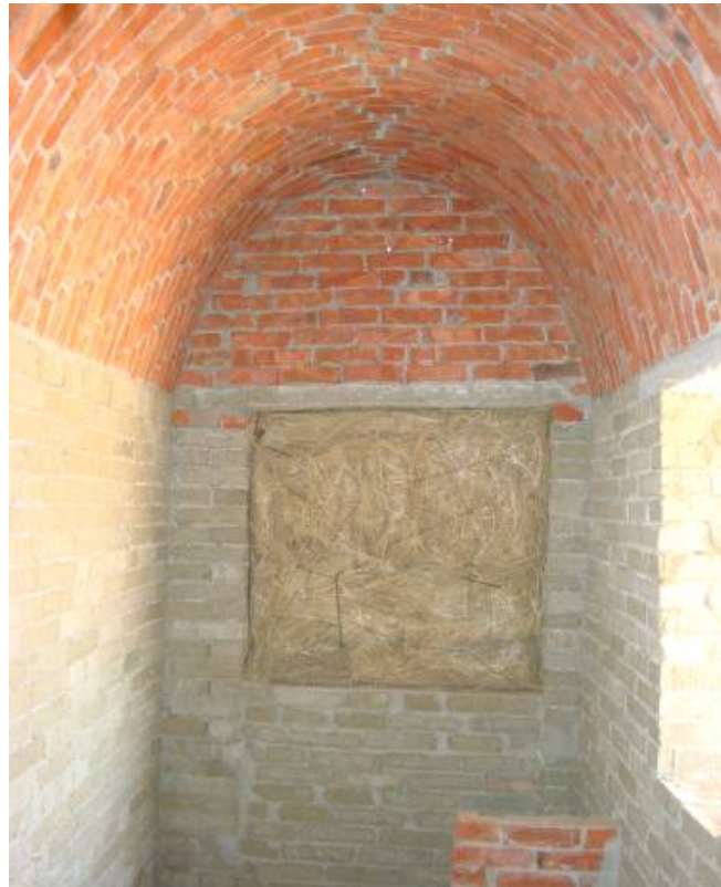
Figure-5. Cementations straw bricks wall supporting the vaults.
