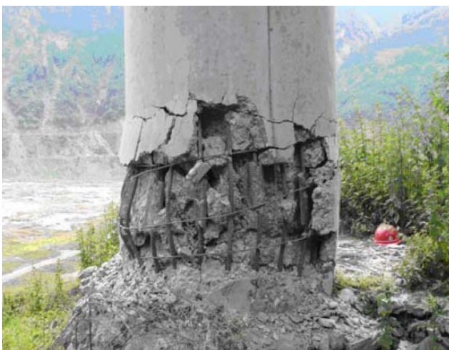
Figure-4. Concrete crusher of pier.
