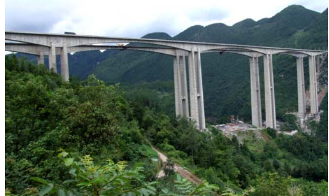
Figure-2. Mashuihe bridge (142m high of pier)
