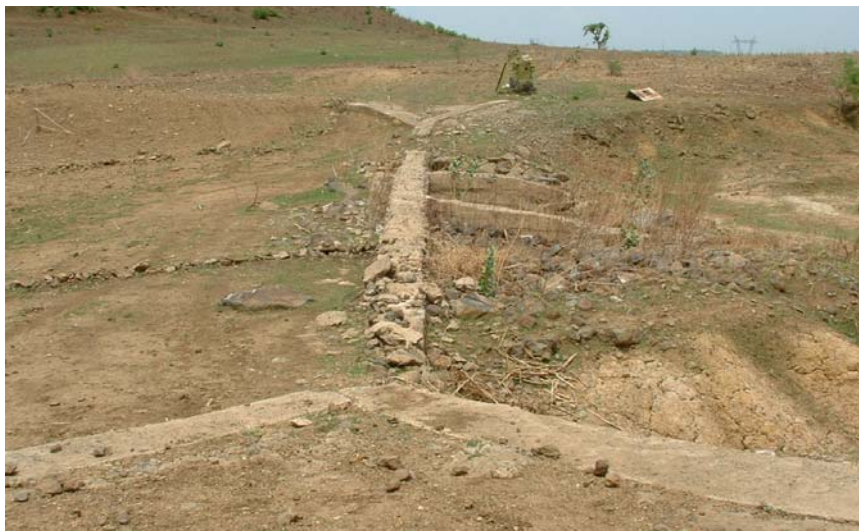
Plate-5. Uncompleted Spill-way.
