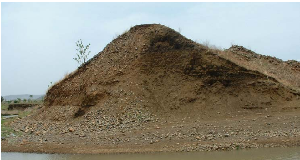
Plate-2. A breached section through the dam shows a uniform material.
