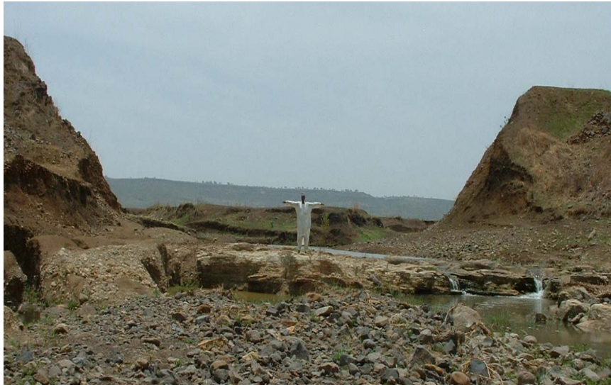
Plate-6. Complete failure of the dam.
