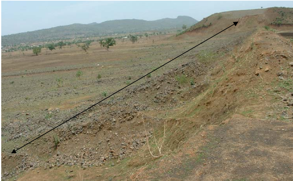
Plate-1. Position of toe weir at down stream covered by rubles.
