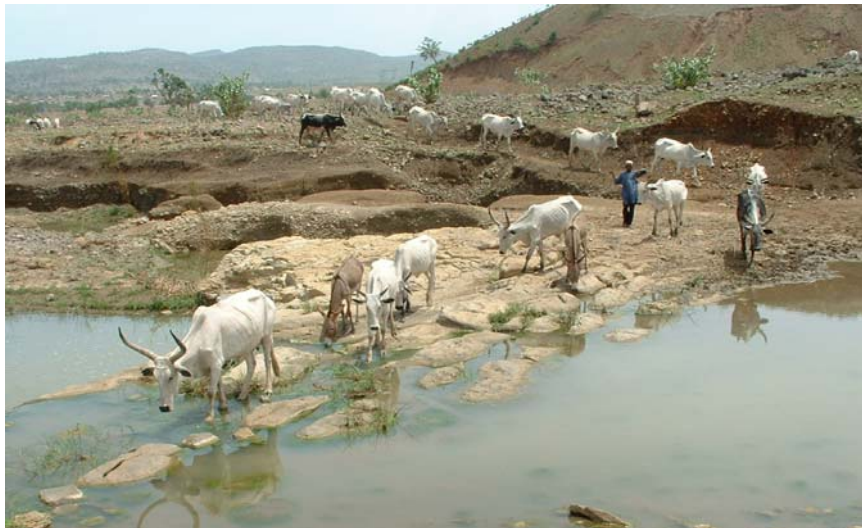
Plate-3. Dam foundation on rocky material not having a key trench.
