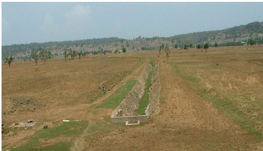
Plate-7. Exit of the Main Canal from the release facility.
