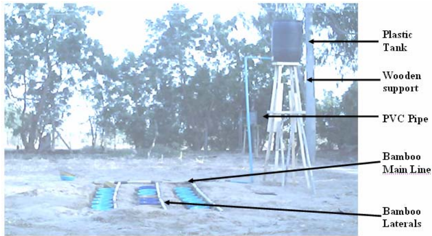
Figure-1. Bamboo micro irrigation system arrangement.
