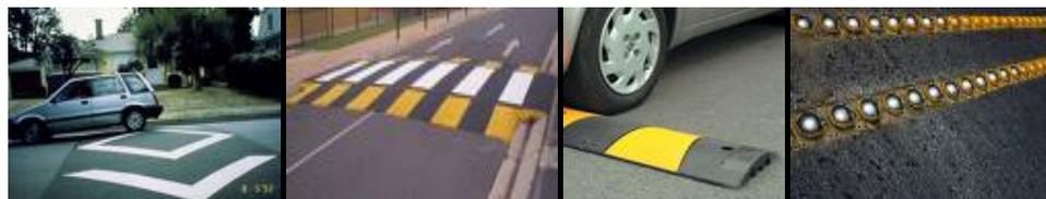
Figure-11. Different designs of speed reducers.
