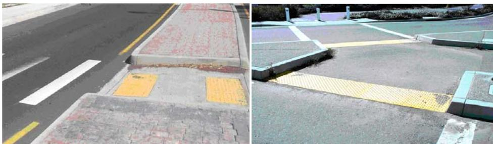
**Figure-6.** Sidewalks and crossing ramps.
