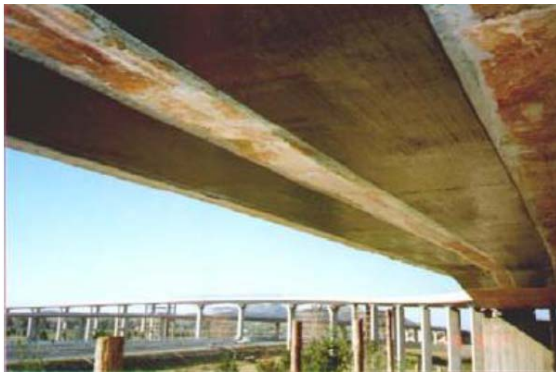
Figure-1. Flexural strengthening of a highway RC bridge slab, China.
