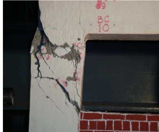
Figure-12. Crushing of the loaded corners.
