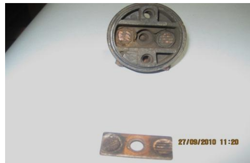
Figure-6. Pitting in hold-in winding contact.
