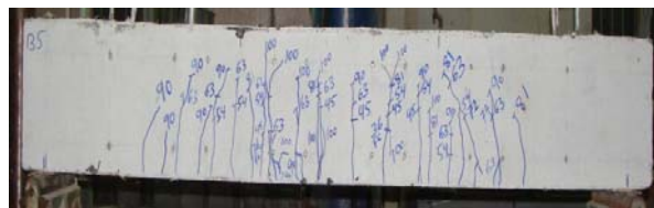
(g). Failure mode for beam ( D_{250}V_{1c} )
