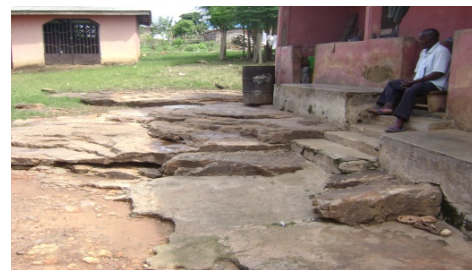
Figure-12. Eroded topsoil in the sumampa catchment.
