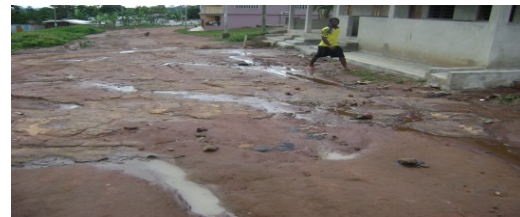
Figure-10. Eroded topsoil in the sumampa catchment.
