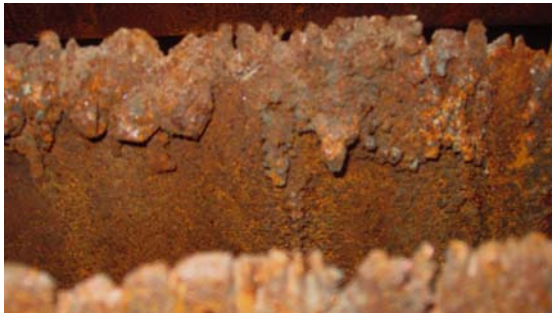
Figure-2. Magnified view of the corroded part.
