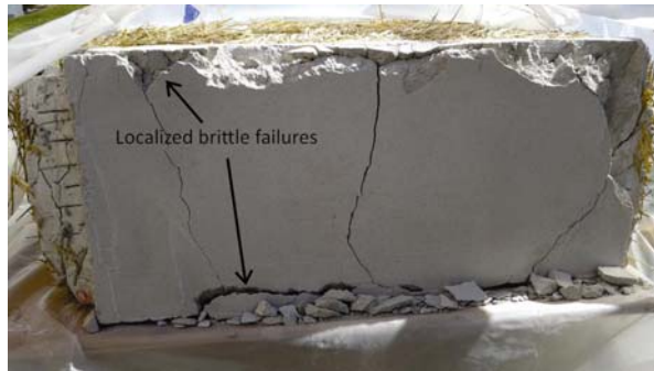
Figure-5. Brittle failure of lime plastered specimen loaded flat.
