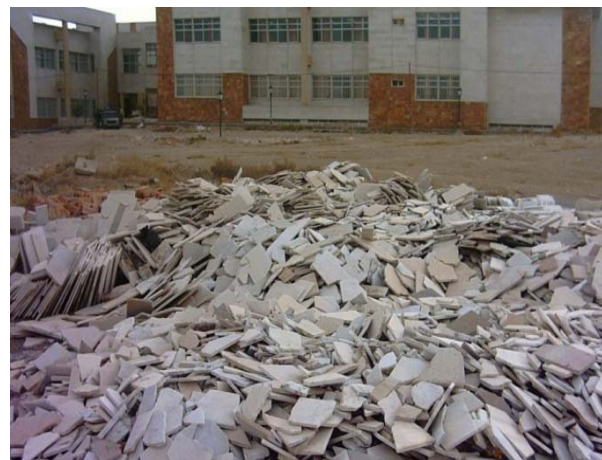
Figure-4. The waste of facade stones due to particular architectural designs.
