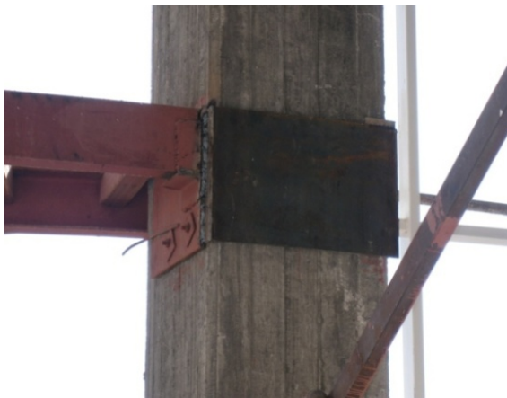
Figure-6. Presenting no implementation details on linking a beam to the pillar.
