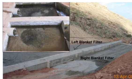
Figure-7. Blanket filter and v-notch chamber at Hamamuk dam.
