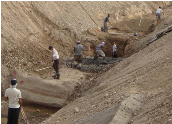
Figure-15. Foundation treatment of bottom outlet gallery at Bawashaswar dam.
