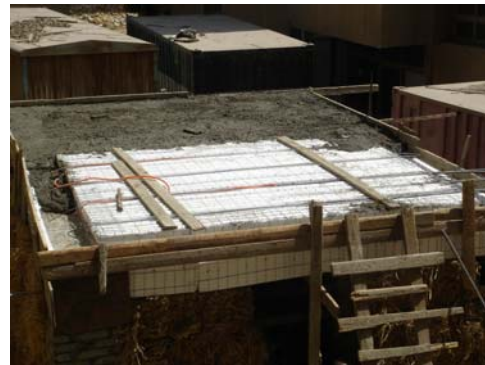
Figure-2(a). M2 System for ground floor slabs and beams.
