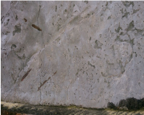
Figure-3. First crack formed in specimen.
