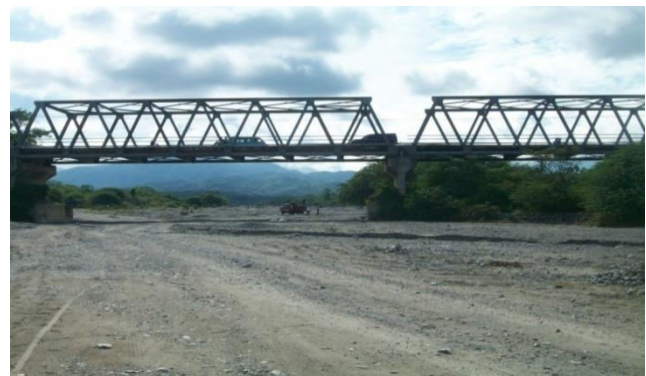
Figure-3. Photos of Taipa bridge from downstream to upstream.
