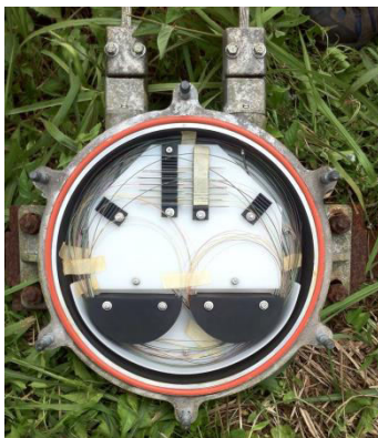
Figure-1. Bending of the optical fibre in joint closure.
